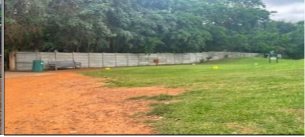
New wall at Hole 15 tee box
