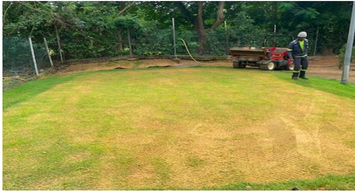
Driving Range Green under construction
